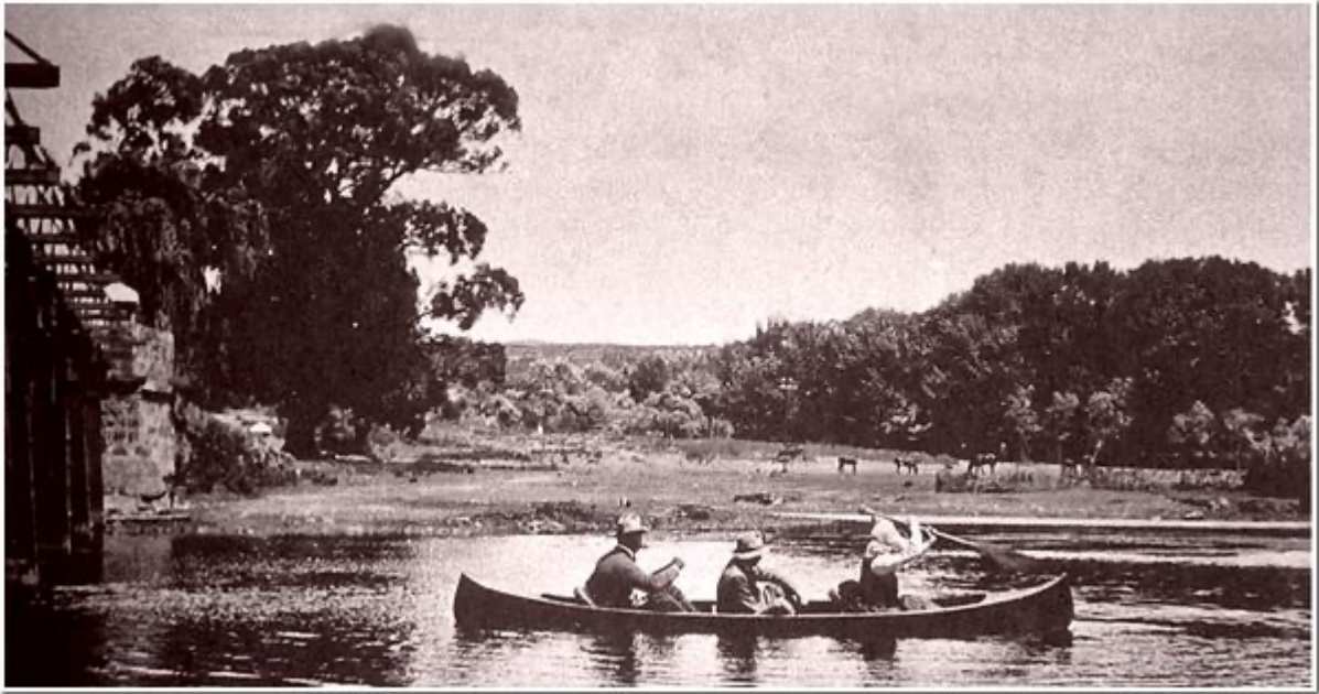
WEIR AT GRABOUW BRIDGE
